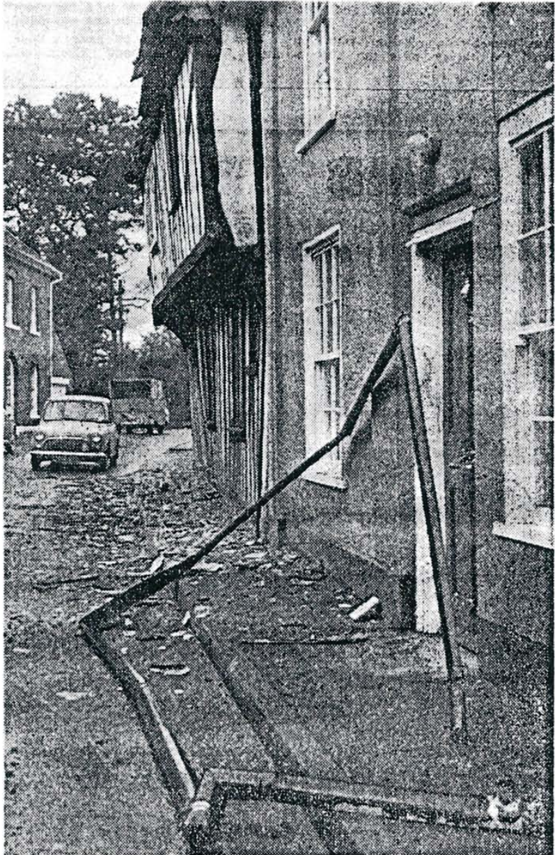
Guttering was torn from the former public house in the accident.
