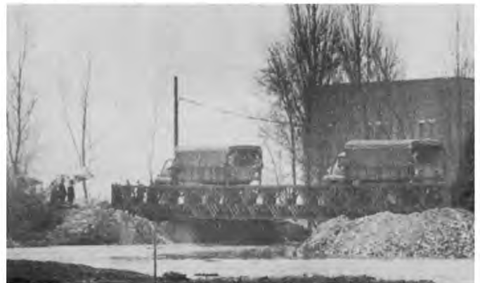
Royal Engineers erecting the Bailey bridge across the Stour, and below testing it with their lorries.
